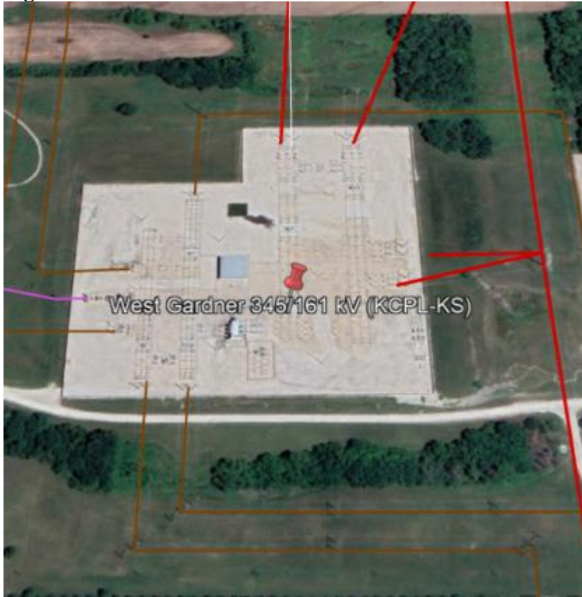
Figure 24 – West Gardner 345kV substation
