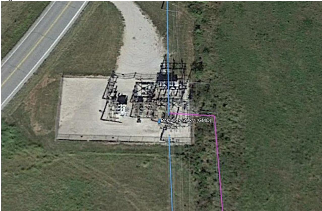
Figure 4 – Post Oak – 69kV Transformer
