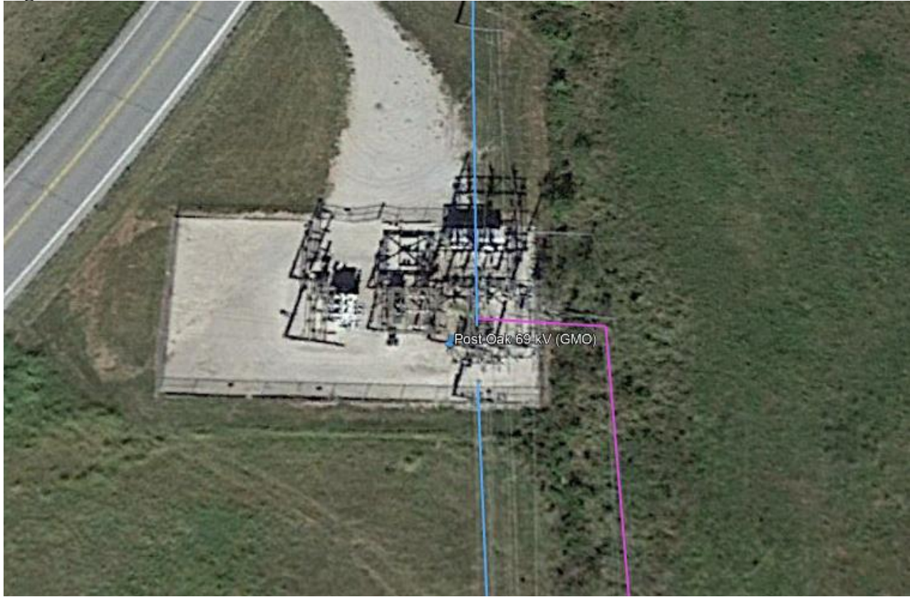
Figure 4 – Post Oak – 69kV Transformer
